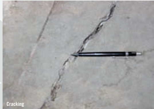
Cracking
